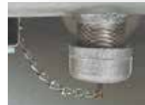
A stainless chain secures the threaded cap for 1-1/2" pipe drain.
